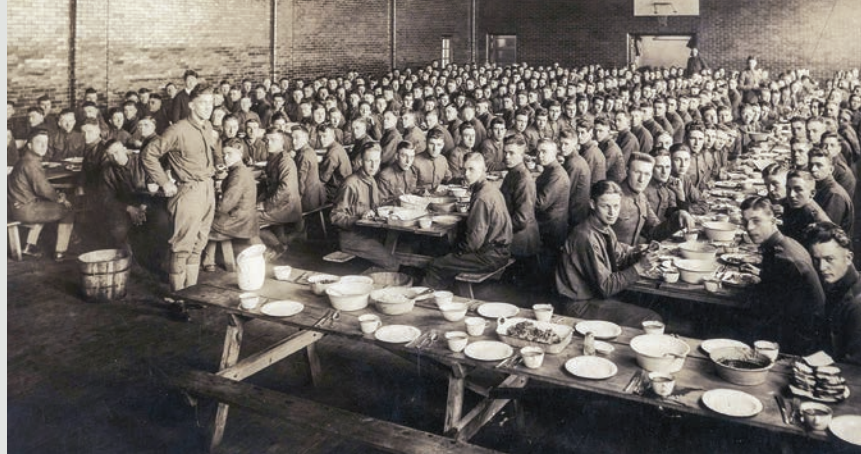
SATC unit in the Mess Hall on the second floor of the new Armory.
